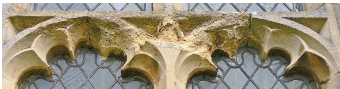
“paid to the stone cutters for mending of church windows ... £0/11s/0d”
